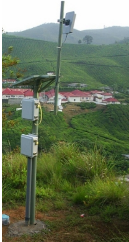
Fig. 8. C3 Sensor Column of Main Deployment
